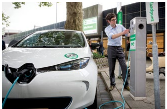
Charging infrastructure in operation
